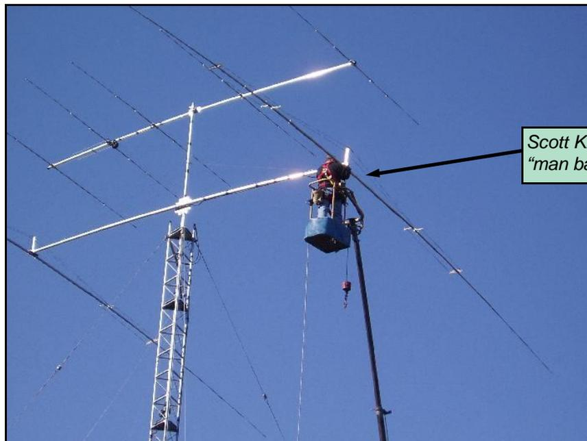
All worked well for 4 days then once again the SWR went to 5:1 all the way across the band. So another call was made to Don K8OMO and back up I went. After checking the connections and with the help of Bill N8PW the problem was traced to a bad coax connector. (bad ground connection).
